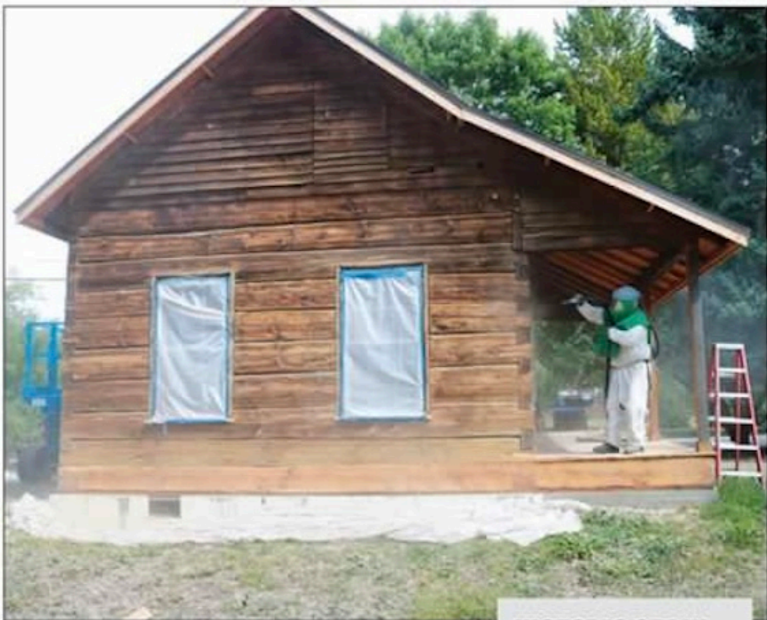
The Colville Indian Agency Cabin gets its new blasting, stain and clear coat thanks to efforts from the community. K.S. Brooks photo
